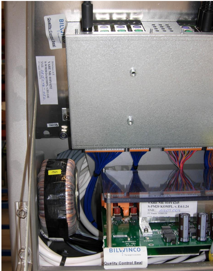
Figure 4. Sealing of boards
