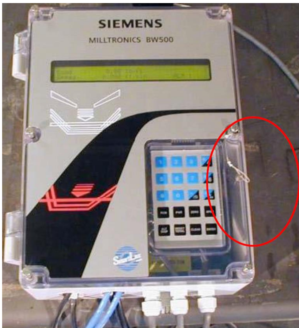
Figure 8 Sealing of BW500
