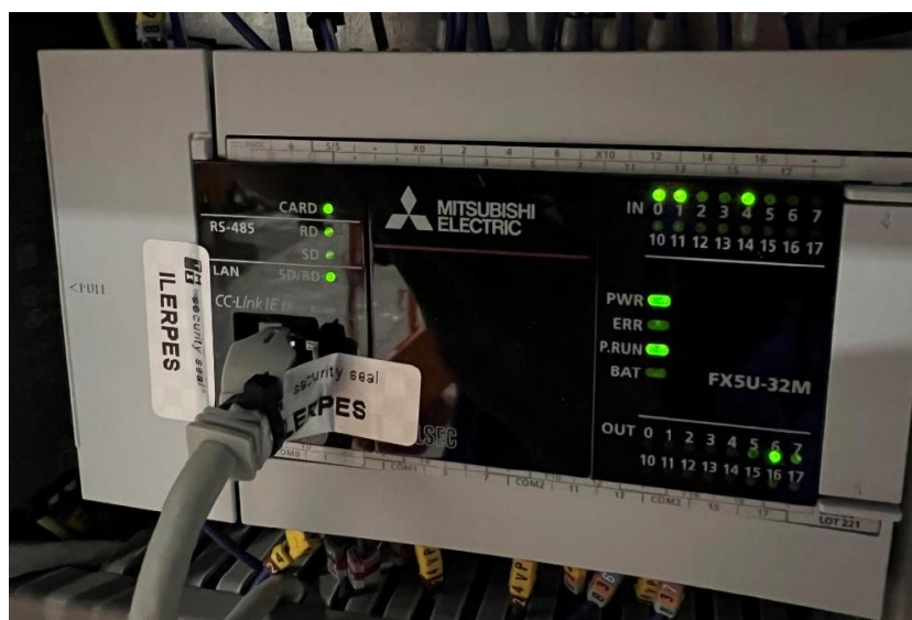
Figure 9. Sealing of the memory card and communication terminals of the FX5U PLC
