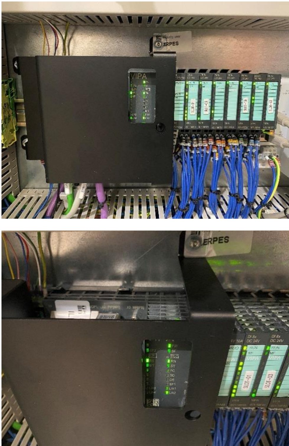
Figure 5. Sealing of LDU 78.1 weighing transducer, the memory card of the PLC and the access to communication terminals of the PLC by a sealed protective metal cover.
